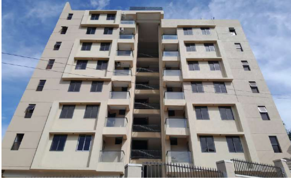
KRISH ROSETTE BLOCK A - NAGURU (Completed)
